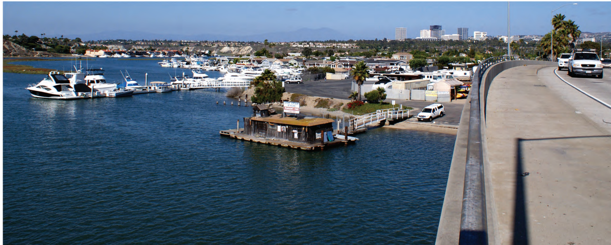
Site Photo from Bay Bridge
